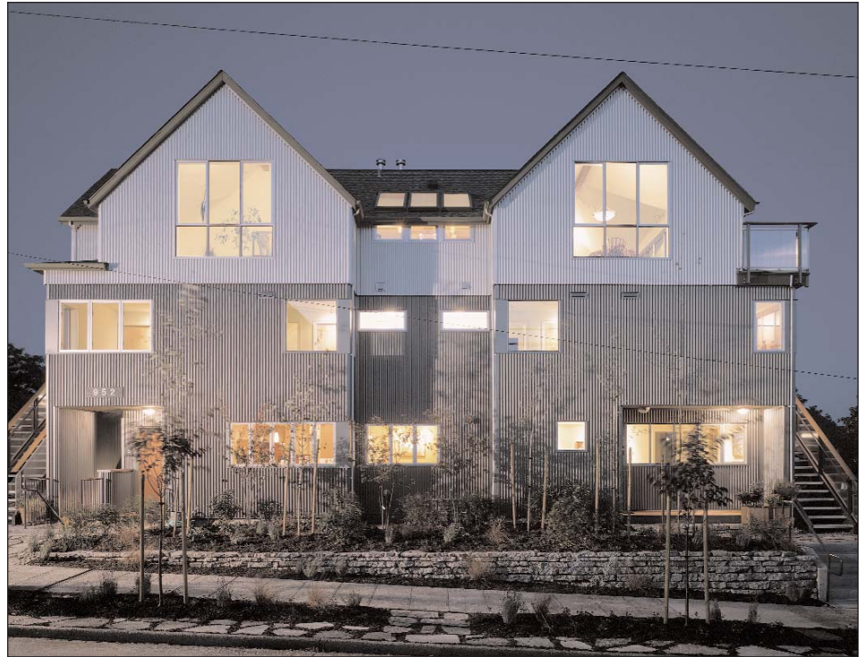
The flats at 42nd Street Condos have large windows and individual entrances. The top units have views of Lake Union and Mount Rainier.
