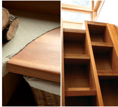
Carpenter Korben Mathis filled the house with well-crafted touches, such as fitting a wooden bench to the shape of stone behind and building a ship's-ladder stairway to the third-floor aerie.
